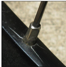
spoke hole cracking
